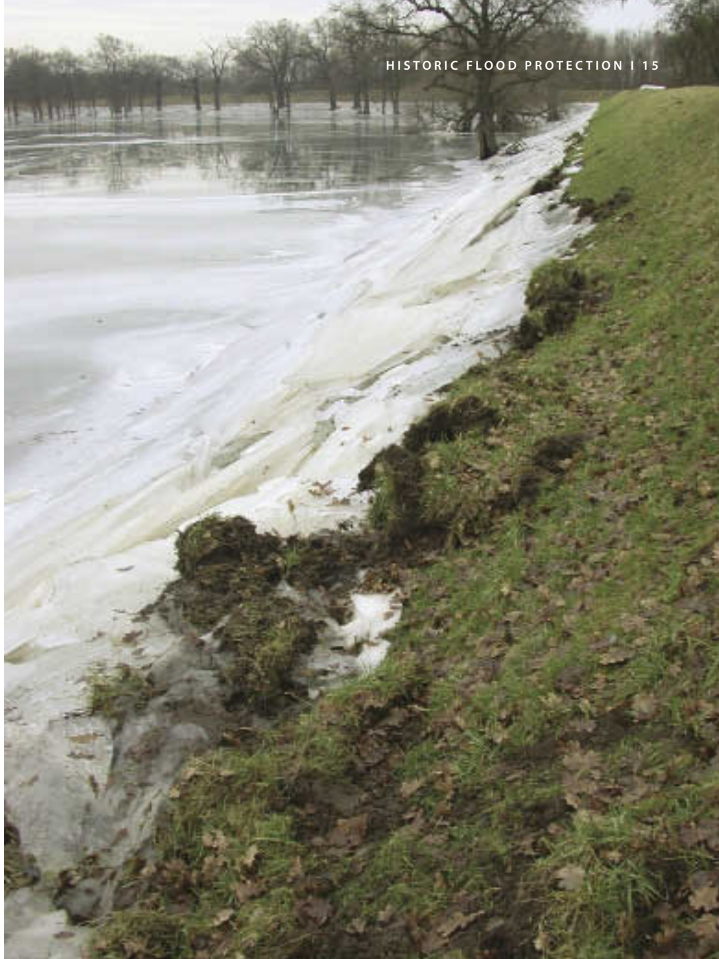
Ice drift and its power to destroy a dyke
